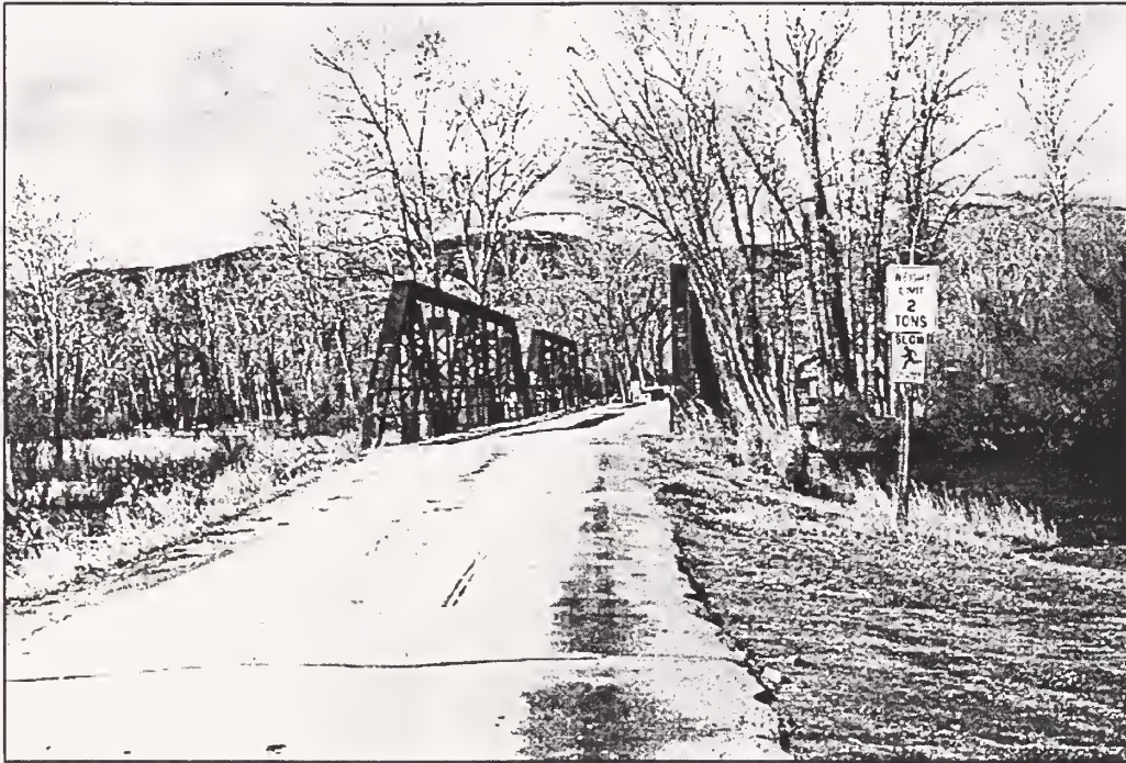
Looking West Across Bridge from East Approach
